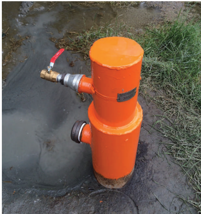
Photo 1. Example of a newly constructed flowing artesian well with multiple casings
