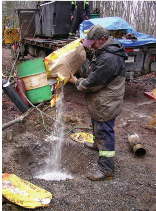
Photo 1. Filling of the well with bentonite chips during decommissioning
